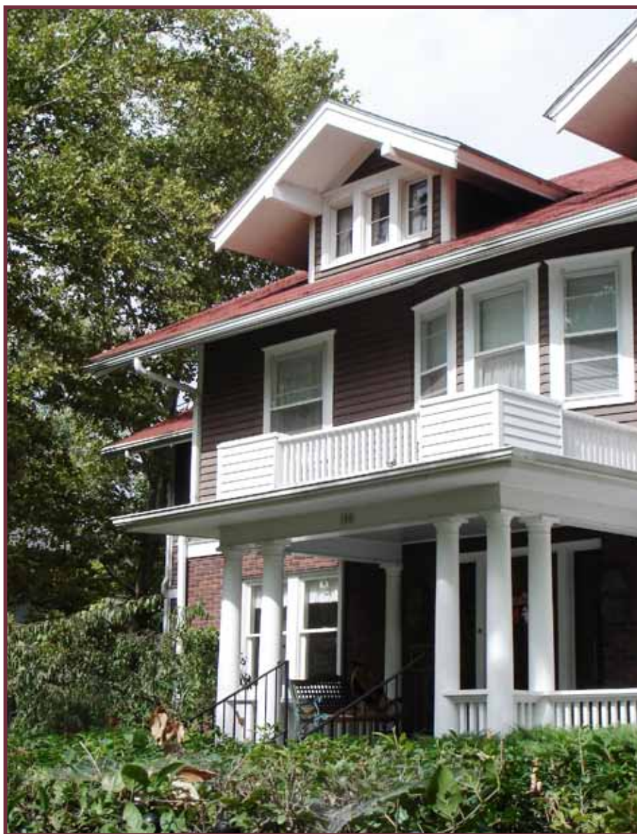
Frank and Dora Wolcott House, Hutchinson, Kansas
