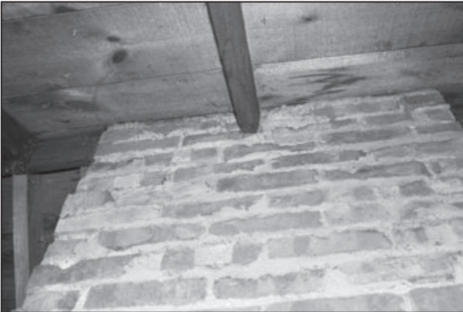
*Chimneys can be a source of air leaks.*
