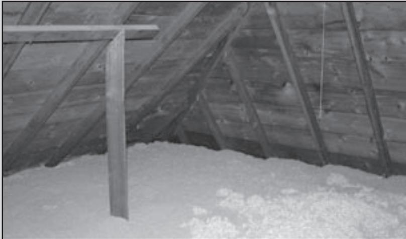
*Cellulose insulation, made from recycled materials, is a good choice for insulating unoccupied attic space.*
