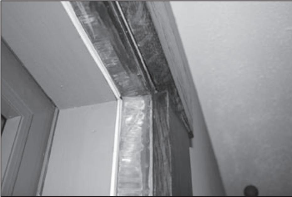
*Weatherstripping keeps air from penetrating gaps around window and doors.*
