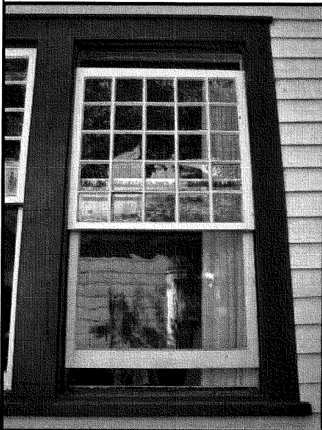
Below: The moveable upper and low sash in traditional double-hung windows draw heat out of the house and let cool breezes in. NAPC file photos
