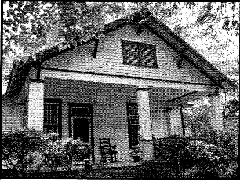
Above: Wide eaves and deep porches were designed to manage the sun in both the summer and winter.
