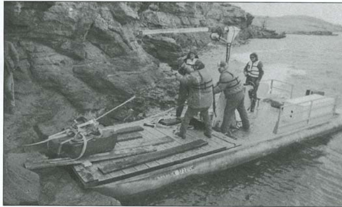
Personnel from the Corps of Engineers staff at Wilson Lake and from the Kansas Department of Wildlife and Parks winch the stone block onto a Wildlife and Parks pontoon boat.
