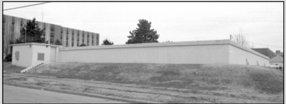
Figure 3 – Waterworks (Black & Veatch Engineers, Kansas City), PWA 1935-36, Pittsburg, Crawford County.
