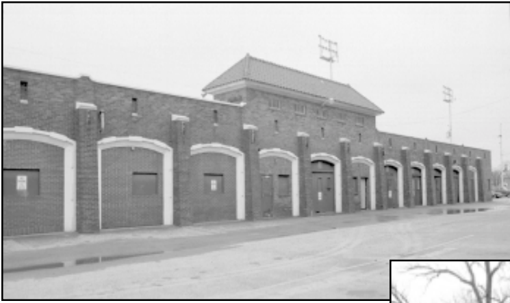
(Top) Figure 6 – Athletic Stadium, WPA 1940, Theodore Roosevelt Middle School, Pittsburg, Crawford County.
