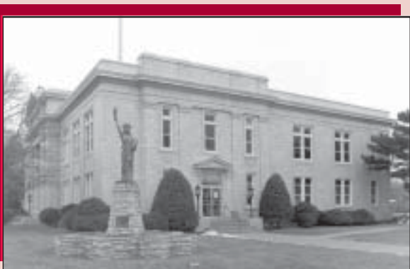
The City of Leavenworth is currently renovating the Leavenworth City Hall and reversing some of the 1970s changes. State tax credits will be used to partially reimburse the City's expenses.
