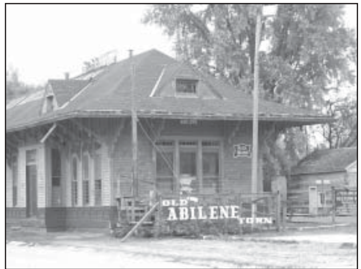
The very wide eaves of the Abilene Rock Island Depot not only provided protection from inclement weather but also served as an area for elaborate decorations, including stick work brackets and carved vertical siding. Here the office bay is incorporated beneath the eaves of the main roof. (This depot has been relocated.)
