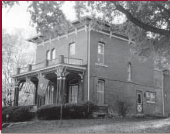
The four fireplaces and two chimneys in this Italianate house located in the Third Avenue Historic District in Leavenworth were rehabilitated through the state tax credit program.
