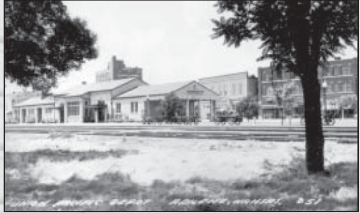
Shown above is a 1935 view of the Abilene Union Pacific Railroad Passenger Depot. The Spanish Colonial Revival style structure was built in 1929 from plans prepared by Gilbert Stanley Underwood, who designed a number of facilities for the Union Pacific between 1924 and 1931.
