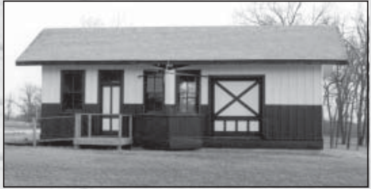
The Bancroft Kansas City and Northwestern Depot is an example of a very simple combination depot, with the office bay formed by two angled walls and incorporated beneath the eaves of the main roof. (This structure has been moved a number of times and is now a museum in Bancroft.)
