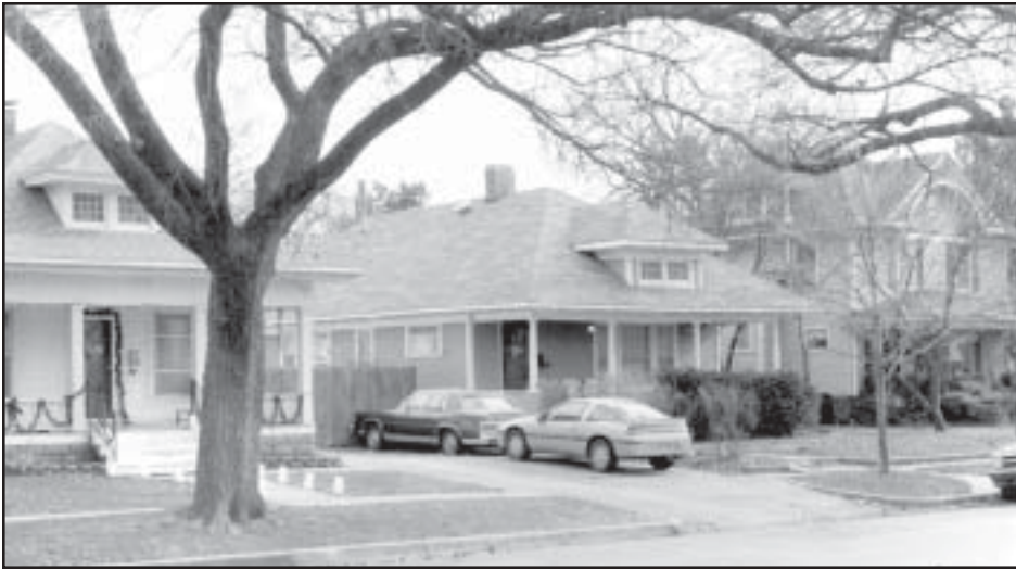
These three residences in the Bitting Historic District, Wichita, demonstrate the variety of late nineteenth and early twentieth century architectural styles and influences present in the district. Located in the 1100 block of North Bitting, they have been identified (left to right) as (1) National Folk; pyramidal; (2) Craftsman bungalow; and (3) Foursquare with Colonial Revival influences.
