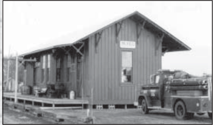
Paxico's 1895 Rock Island Depot, which has been relocated to the Mill Creek Campground, is an example of a small Rock Island combination depot. The roof of the office bay is separate from that of the main building.
