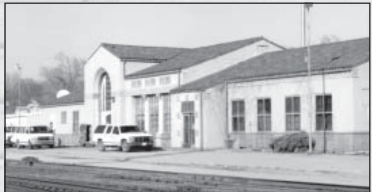
Typical of the attention often accorded to passenger depots, the Marysville Union Pacific Depot is a Mediterranean Revival style example with highly elaborate decorative glazed tiles. Although presently the only crew change point on the Union Pacific line, the railway is relocating the line and this station's future is uncertain.
