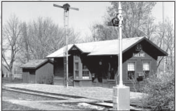
The Pauline Santa Fe Depot was moved to Topeka’s Ward-Meade Park in the late 1970s. The simple combination depot has been nicely restored and maintained by the Topeka chapter of the National Railway Historical Society.
