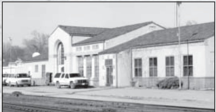
Typical of the attention often accorded to passenger depots, the Marysville Union Pacific Depot is a Mediterranean Revival style example with highly elaborate decorative glazed tiles. Although presently the only crew change point on the Union Pacific line, the railway is relocating the line and this station's future is uncertain.
