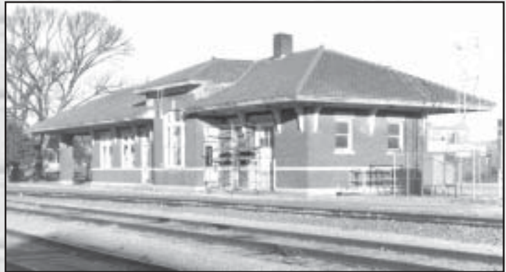
The Downs Missouri Pacific Depot was added to the National Register in 2001. It has been rehabilitated with the assistance of a Heritage Trust Fund grant for use as a community center/museum.
