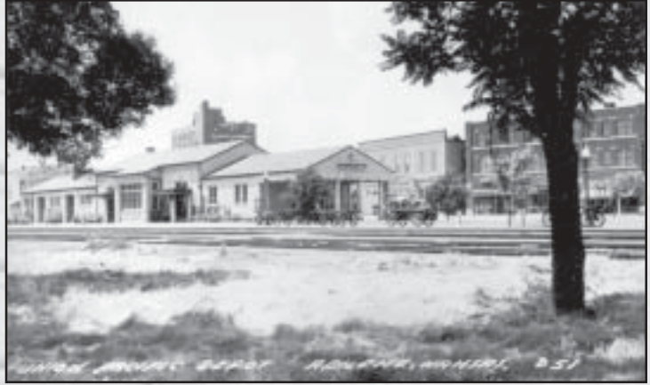
Shown above is a 1935 view of the Abilene Union Pacific Railroad Passenger Depot. The Spanish Colonial Revival style structure was built in 1929 from plans prepared by Gilbert Stanley Underwood, who designed a number of facilities for the Union Pacific between 1924 and 1931.
