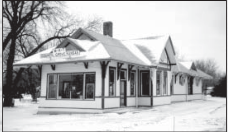
The depot at Council Grove is one of the more elaborate Missouri, Kansas and Texas depots. Listed on the National Register in 2001, it is one of the few remaining KATY depots left in Kansas, and possibly the only one on its original site. It is currently for sale.
