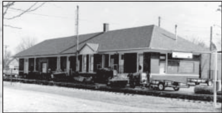
The 1882 Augusta Frisco Passenger Depot originally had a tile roof, but was one of the few buildings in Augusta which survived a 1920s tornado. It may also be the only surviving brick Frisco depot left in the state.
