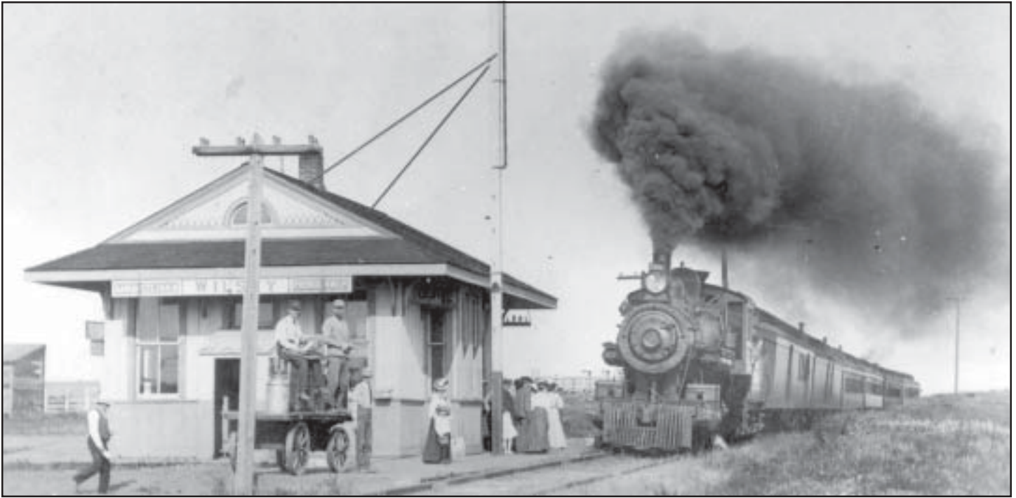
This early twentieth-century photo shows the train arriving at the Missouri Pacific Depot in Wilsey. Although modest in size and appearance, the depot was enhanced by decorative gable ends and the imaginative roof line.
