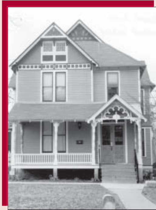
The E. F. Goodrich House in Lawrence was renovated with the assistance of tax credits. The owners converted the 1890 Queen Anne home into offices for their medical practice. The renovations, including general repairs and painting, were completed in December 2002.
