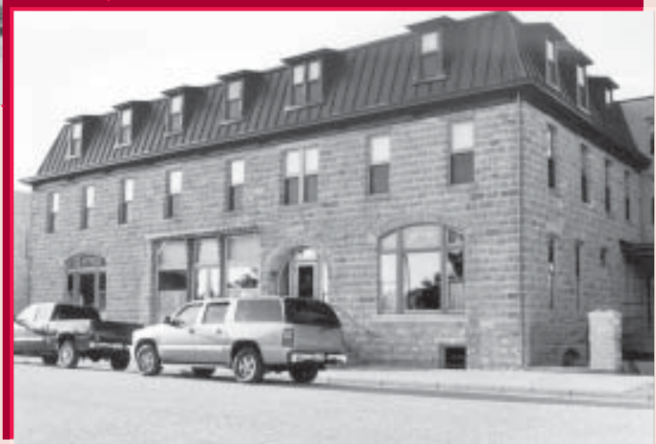
(Right) The owners of the Midland Hotel in Wilson utilized tax credits to return the building to service as a hotel. Modern conveniences were combined with historic features such as stained glass windows, wood floors, and ornate wood trim. The hotel was completed and opened to visitors in the summer of 2003.
