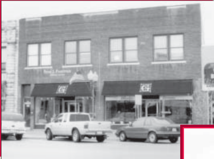
(Left) Rehabilitation work on the Higinbotham Building on Poyntz Avenue in Manhattan was completed in 2002 utilizing tax credits. The building, constructed in 1918, is a contributing element of the Manhattan Downtown Historic District. The rehabilitation involved repair and maintenance work to the roof and exterior masonry along with window replacement and remodeling of the second floor to accommodate offices and apartments. The Higinbotham Building has a furniture and gift store on the street level with offices and apartments on the upper level.
