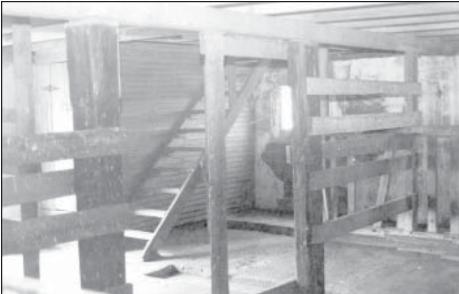
The interior of the ground level is dominated by three rows of five stanchions for dairy cattle; the ground level also features a four-foot by seven-foot grain bin.
